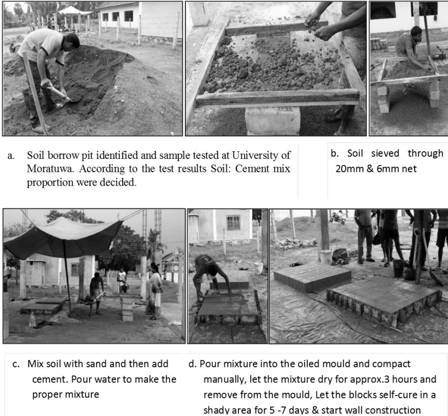
Figure 7: Mud- Concrete block Casting and curing procedure at Site
