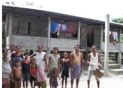
Figure 13 Typical RCC framed house on Stilts
